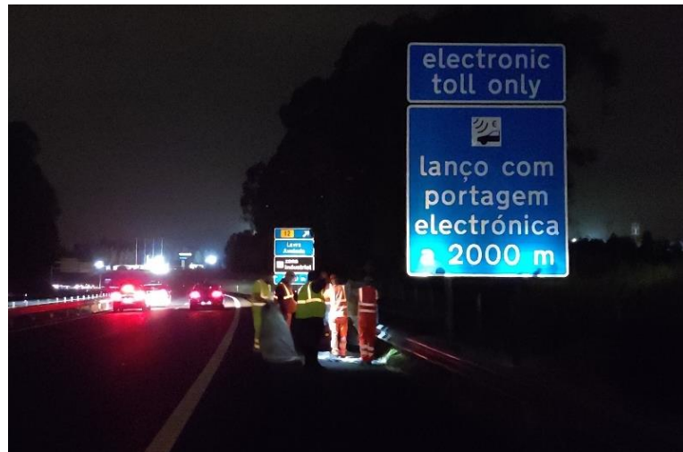
Figure 4: The metal information road panel in A28 ES-PT causes radio signal blocking. This effect was mitigated by covering it with a thick plastic sheet.
