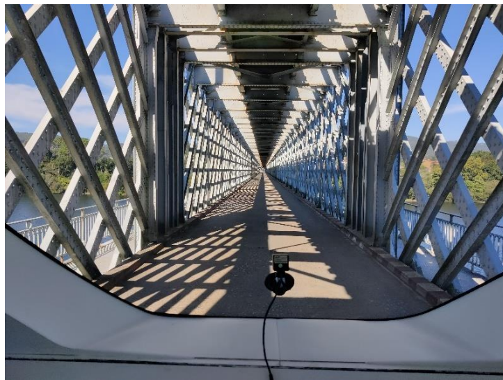
Figure 3: The metal structure of the Old Bridge ES-PT acts as a signal attenuator. This effect was mitigated with the installation of a small cell.
