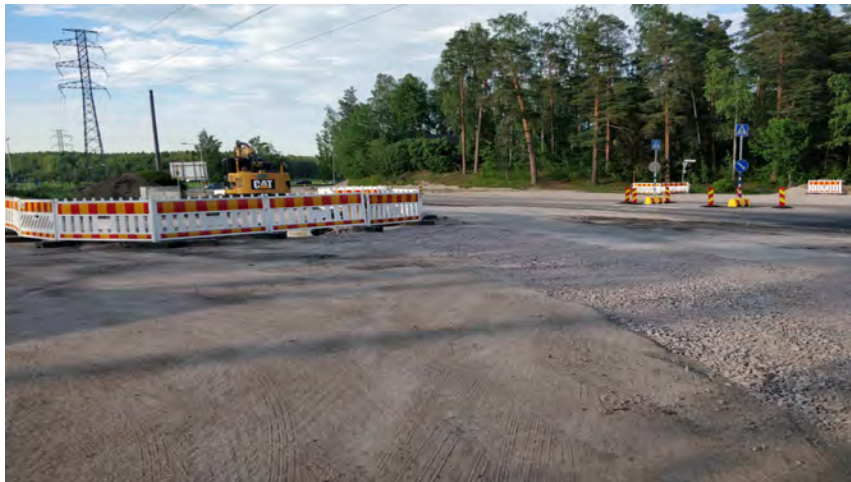
Figure 20: Image with construction work captured in Espoo, Finland.
