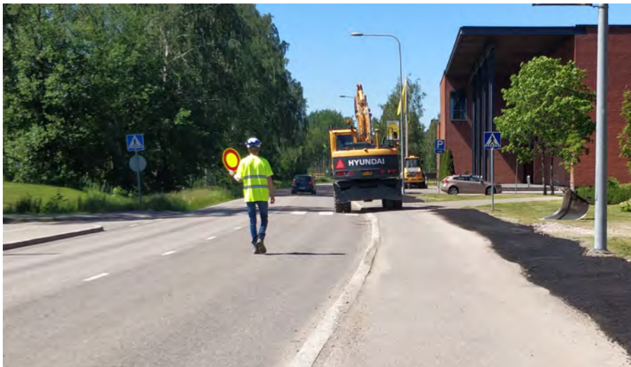
Figure 13: Construction site Finland with a temporary caution sign.
