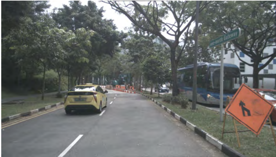
Figure 12: Construction site in Singapore where construction sign is not very clear.
