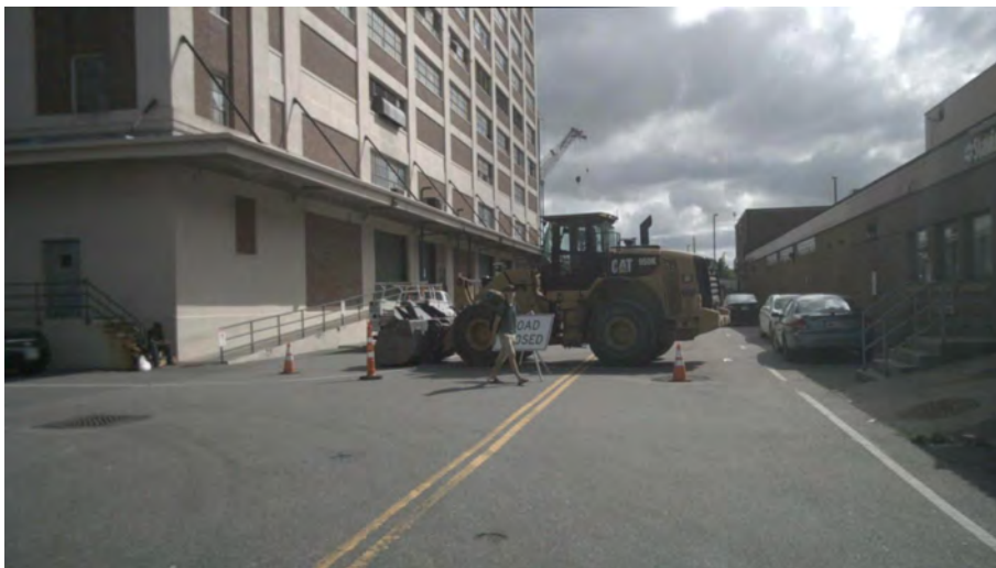
Figure 11: Road closed for construction work.
