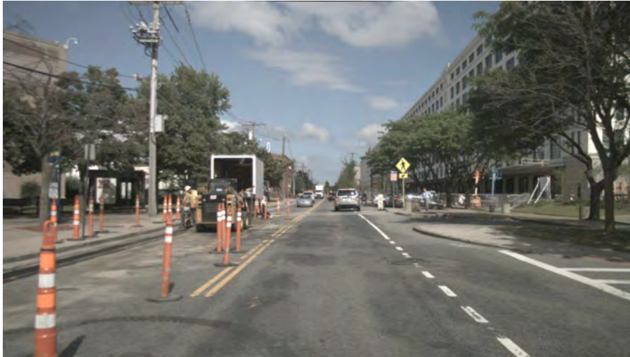
Figure 10: Lane blocked for fixing a pothole.
