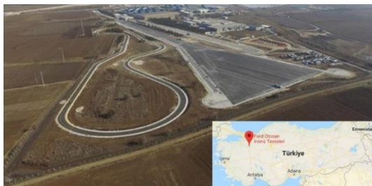
Figure 2: Ford Otosan test site to be used for long-term functionality development and testing
